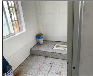
Photo of the sanitary facilities toilet.JPG
